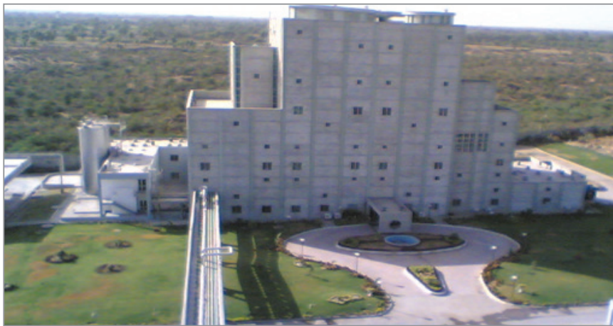
Fig. 1.3.2. Outer view of a large-size dairy processing plant
