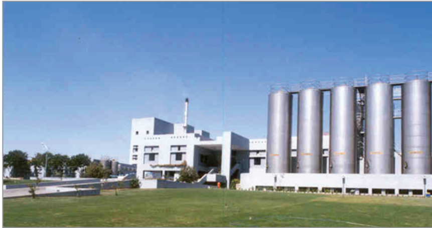
Fig. 1.3.1. Outer view of a large-size dairy processing plant
