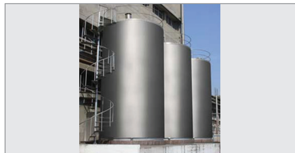
Fig. 3.1.2. Vertical insulated milk storage tank
